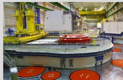
Figure 3 Reactor hall of Mochovce 3.
