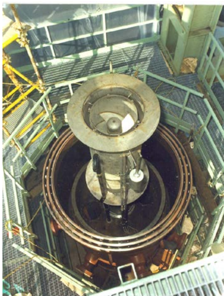
Installation of a 20-inch Steam-Water separator in the GEST-SEP facility vessel
