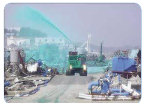
Figure 10 - Decontamination using synthetic resin emulsion (source “TEPCO, WNN”)
