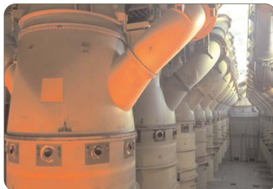
Uranium enrichment cascade based on diffusion technology
